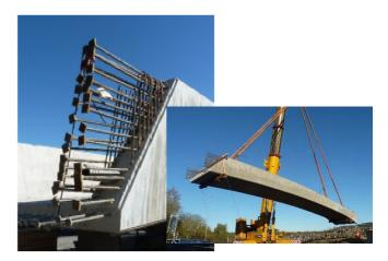
Potential application: lap splice of prefabricated elements. Use of headed bars for short splice length.
