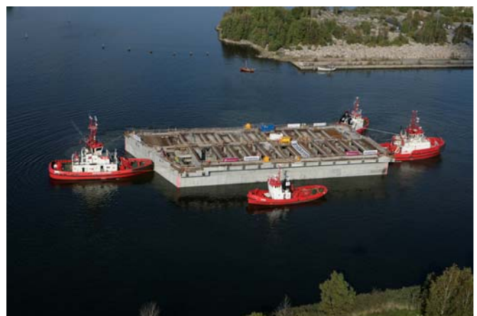
Tow of a concrete caisson to the site (Photo: Skanska)
