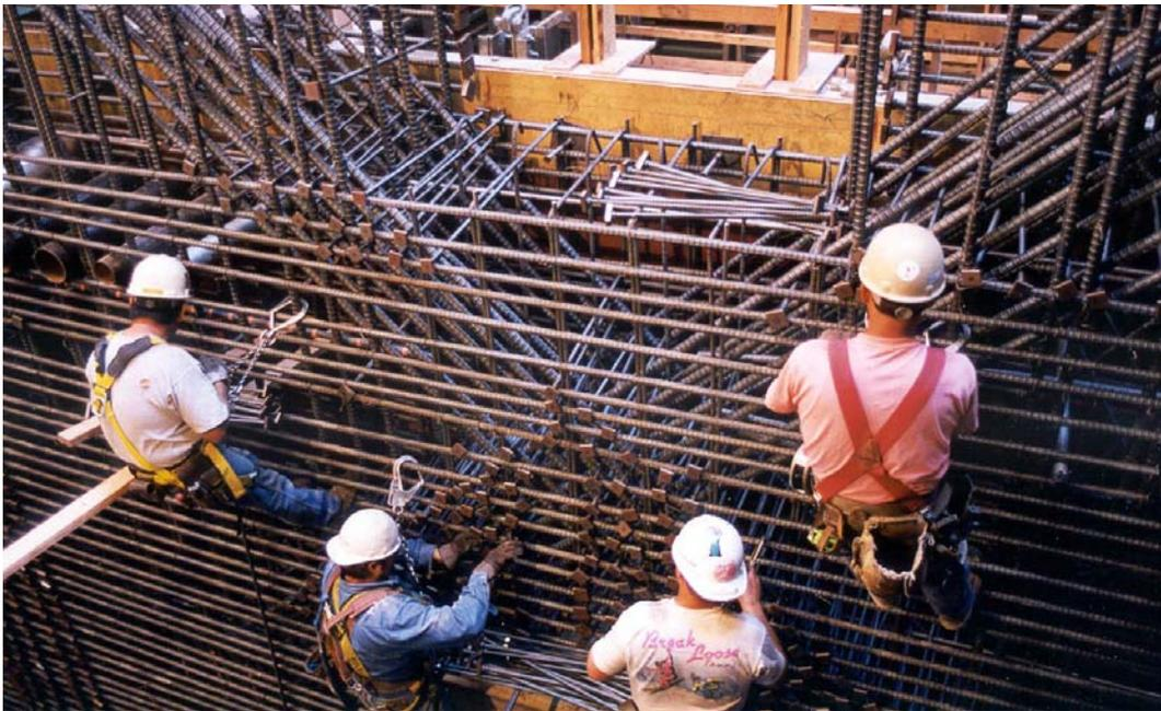
HRC T-headed bars have some special characteristics which distinguish them from conventional reinforcement. HRC T-heads anchor the full actual tensile capacity of the rebar. Thus the reinforcement stays fully anchored beyond yielding up to bar break. That makes it possible to use the real stress- and strain capacity of the reinforcing steel, i.e. the ductility of the rebar.
